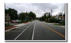
Edge Line Striping: Edge line striping is also effective in residential areas to narrow the lanes and/or provide additional delineation for other uses. Reducing the lane width has the potential for reducing speed by creating a narrower traffic lane. The area between the edge of the road and the lane marking can often be used for parking or as a bike lane, depending on the resulting shoulder width.
