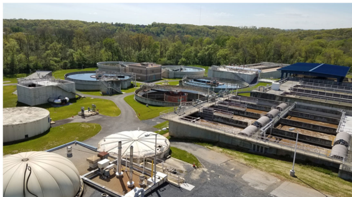
J. Hase Mowrey Regional Wastewater Treatment Facility
